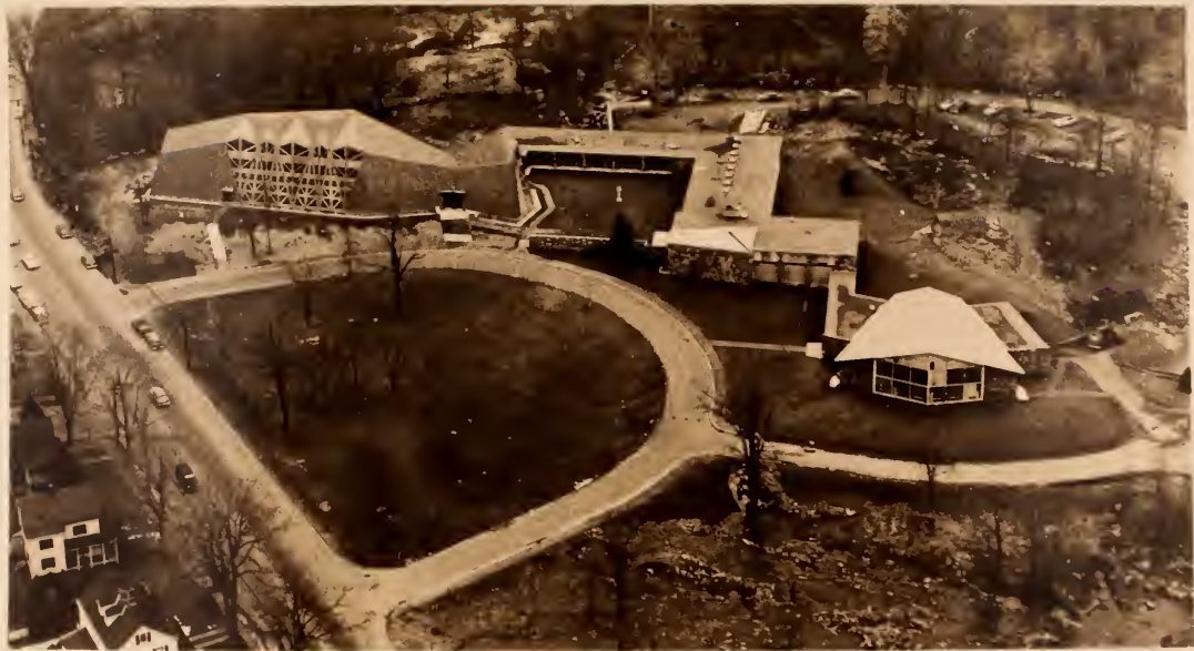
Air View, First Presbyterian Church, Stamford, Conn.
